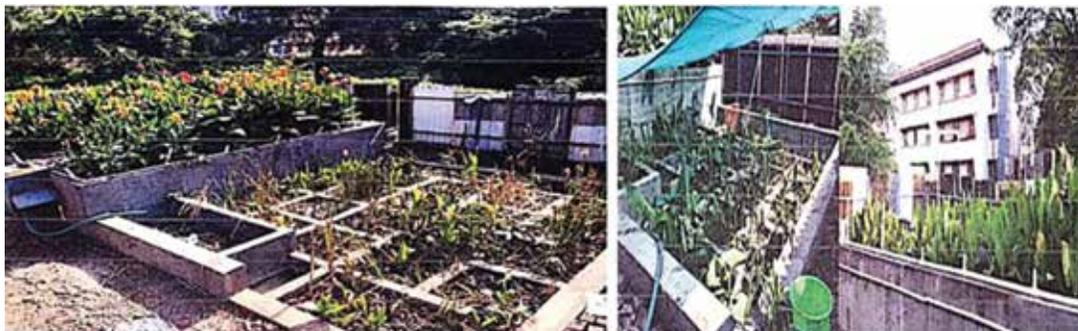
**Figure. 10. Integrated domestic wastewater treatment system with multi-species and dual media constructed wetland**
