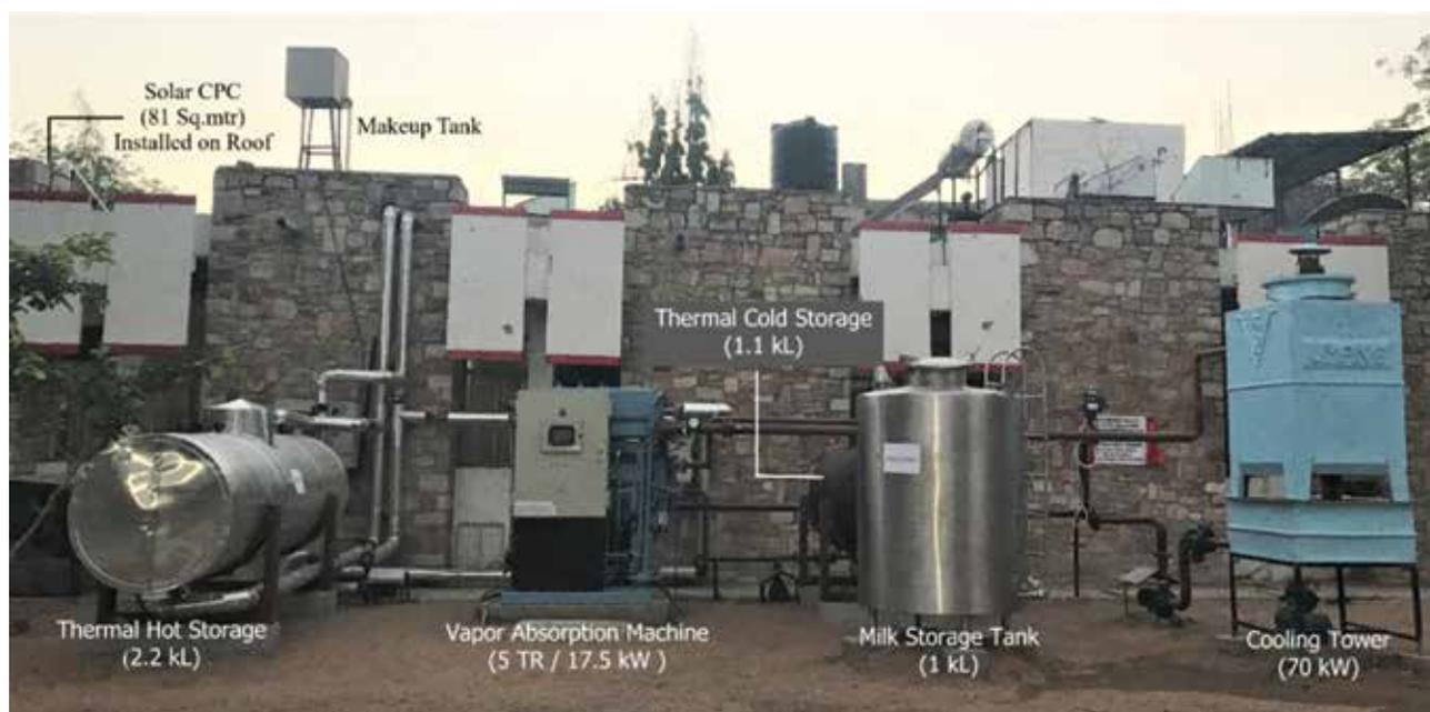
**Schematic of the Solar Thermal Assisted Rapid Bulk Milk Cooler**
